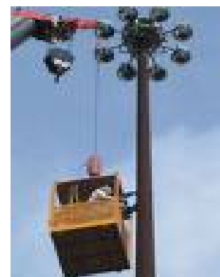
High Mast Lighting Pole
