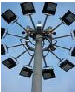
High Mast Lighting Pole
