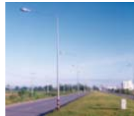
Lighting Pole 9 m.
